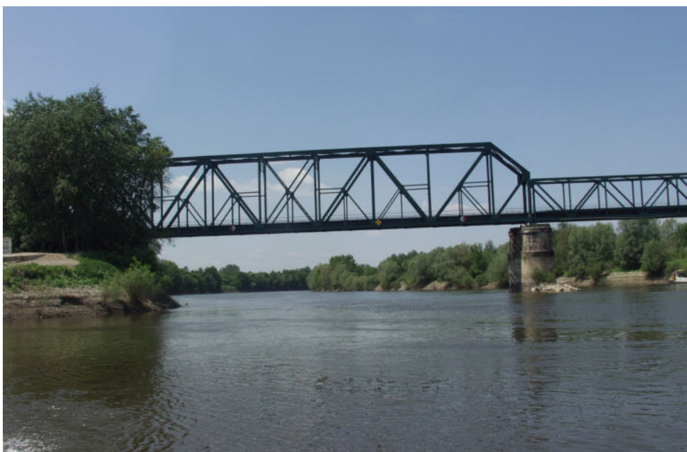
Sl. 43. Jasenovac – željeznički most
